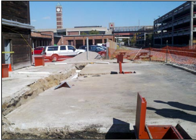
CONVEYANCE PIPE TRENCHING WITH WELL ACCESS VAULTS
