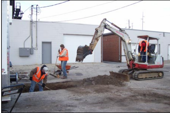
CONVEYANCE LINE TRENCH WORK
