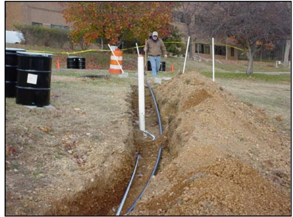
CONVEYANCE LINE TO EXTRACTION WELL CONNECTION.
