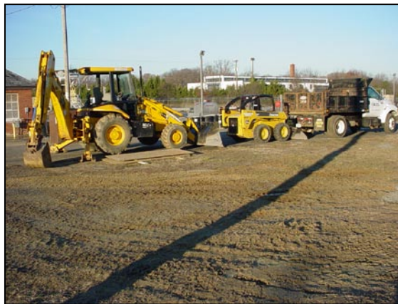
SITE RESTORATION, GRADING ACTIVITIES.
