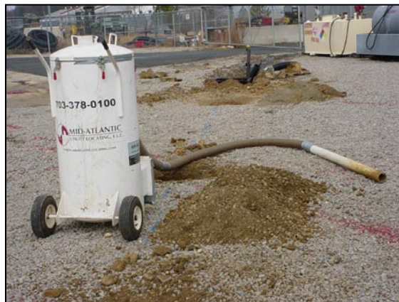
PRE-EXCAVATION UTILITY EXPOSURE, AIR-KNIFING.
