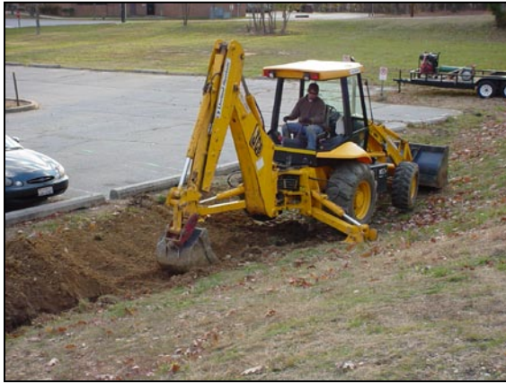
SUBSURFACE CONVEYANCE LINE TRENCHING.
