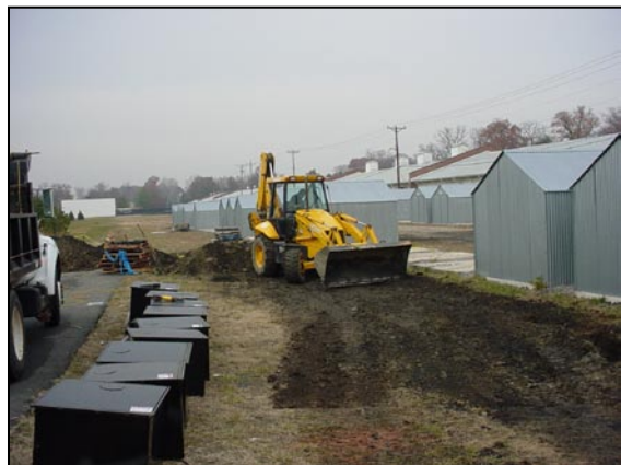
GRASSY AREA BACKFILLING.
