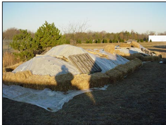
ON-SITE STAGING OF POTENTIALLY IMPACTED SOILS.
