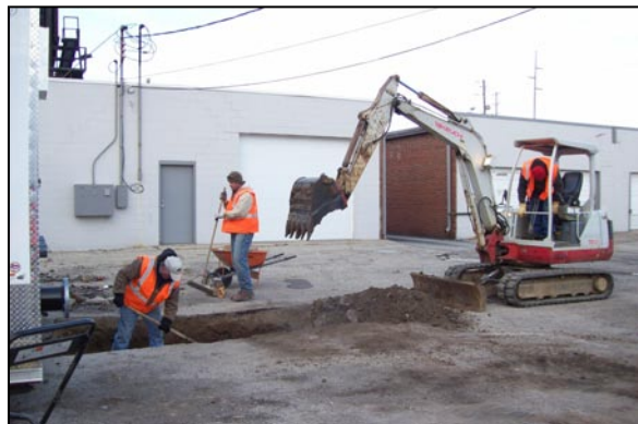
CONVEYANCE LINE TRENCH WORK
